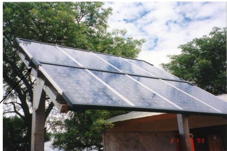
Detail of security frames enclosing modules onto structure
